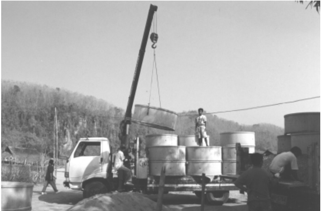
A truck delivers well rings to a village that was forced to relocate to the flat lands.
