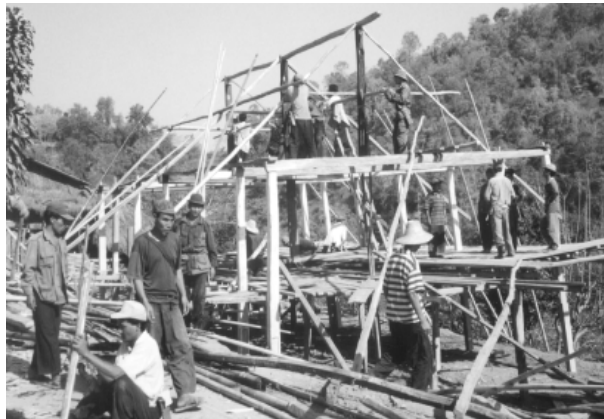
Villagers building a new house
